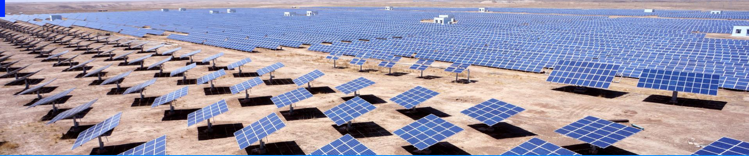
China Republic 100MW Tracking + Ground Mounting
