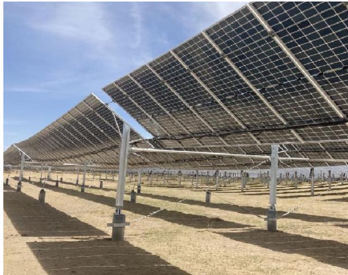
150MW Flexible Mounting In Hainan, China
